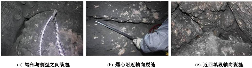
(a) 端部与侧壁之间裂缝 (b) 爆心附近轴向裂缝 (c) 近回填段轴向裂缝
