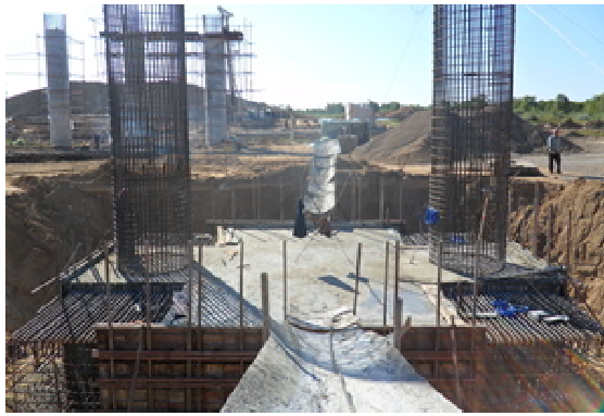
图3 封桩前承台外观
